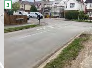
Dropped kerb at the Boyslade Road / Sketchley Road junction
