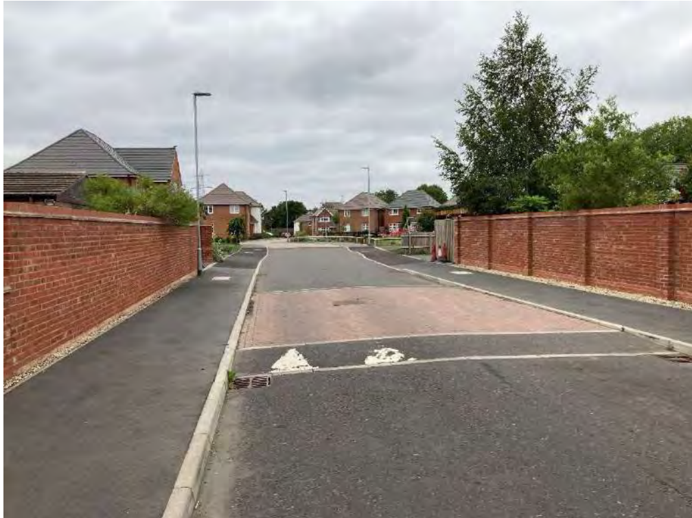
Photograph 3: Passchendaele Drive Facing Westbound
