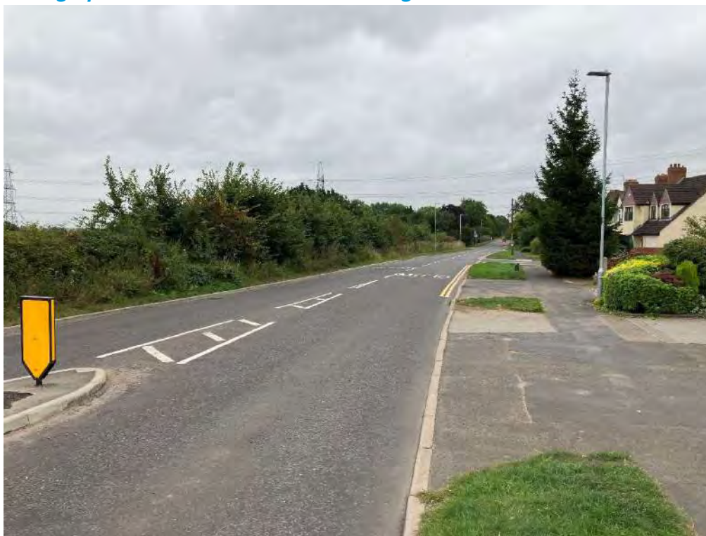
Photograph 4: B578 Lutterworth Road Facing Southward
