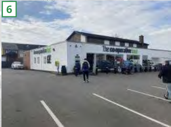
Co-op from the footway at the Boyslade Road / Tilton Road junction
