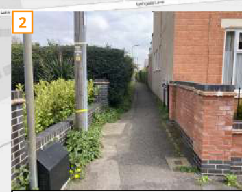
U81 Footpath from Workhouse Lane to the B578 Lutterworth Road
