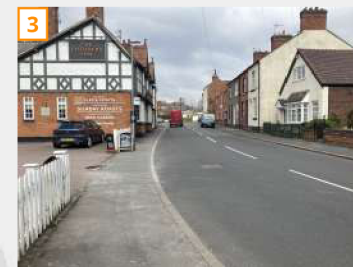
Footways along the B578 Lutterworth Road facing north
