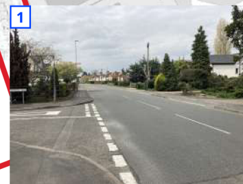
Dropped kerbs and 2m footways along Coventry Road
