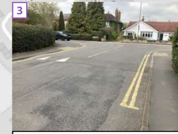
Tactile paving and dropped kerbs at Salem Road / Grove Road junction
