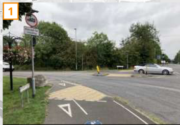
Dropped kerbs and tactile paving at the 3m shared footway / cycleway along the B4109 Rugby Road
