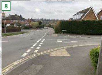
Dropped kerbs and tactile paving at junction
