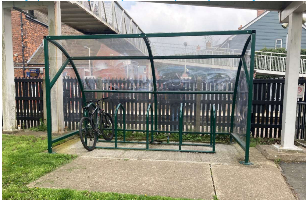
Photograph 1: Hinckley Railway Station Platform 2 Cycle Parking
