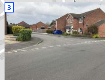
Dropped kerbs at the Pyeharps Road / Grange Drive junction
