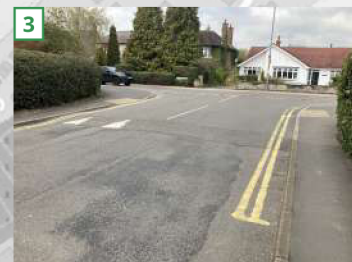
Tactile paving with dropped kerbs at Salem Road/Grove Road junction
