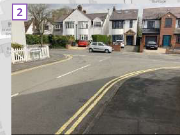
Dropped kerbs at the Salem Road / Victoria Road junction
