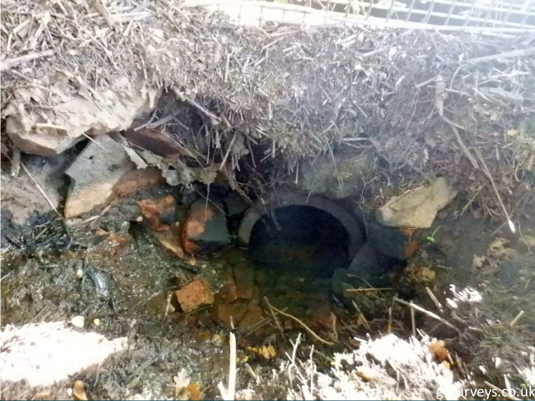
Upstream face, looking downstream
