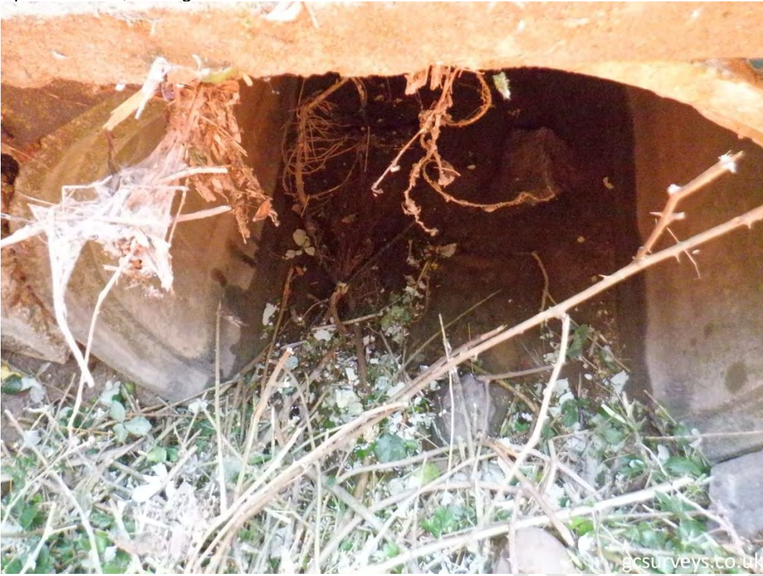
Upstream face, looking downstream.
