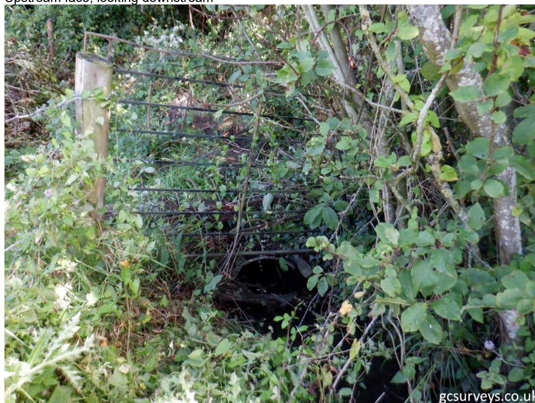
Upstream face, looking downstream
