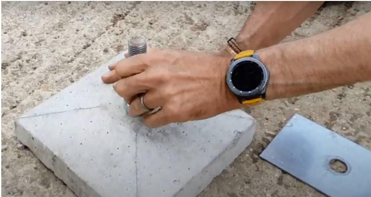
Pad foot for spreading load over ground
