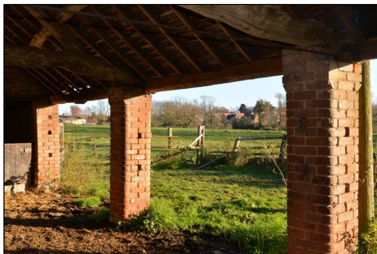
Brick piers to the south elevation showing brick detailing, looking south-east Fig 14
