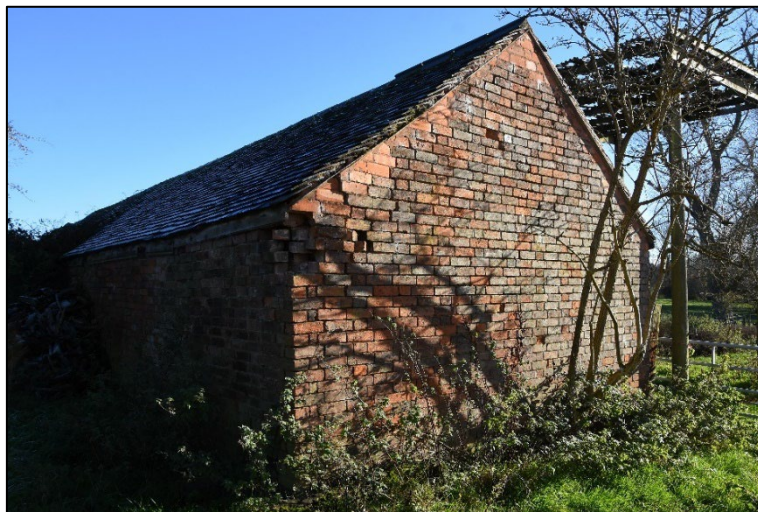
West gable end of the building, looking south-east Fig 16
