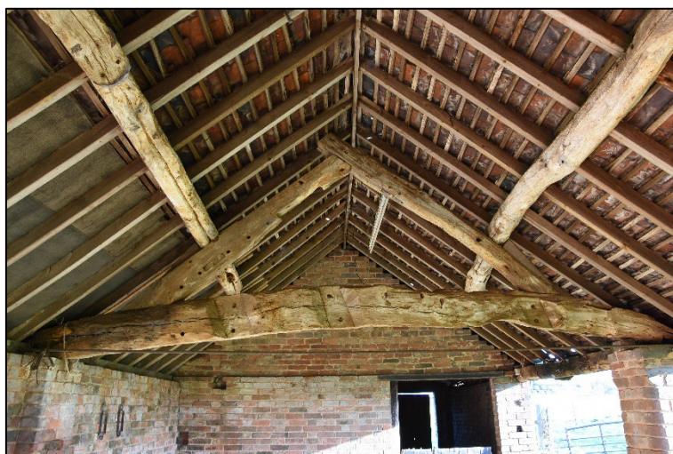
West side of Truss 1, looking east Fig 20
