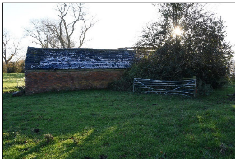
North elevation of the building, looking south
