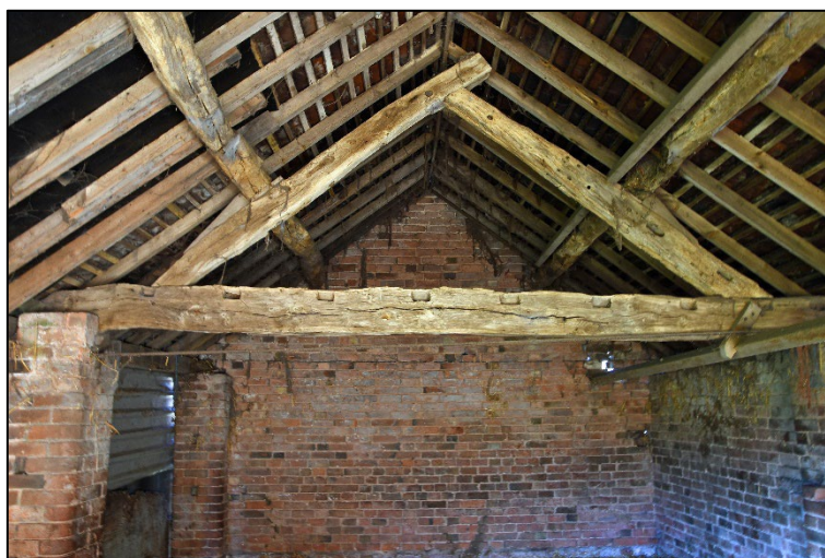
East side of Truss 4, looking east Fig 26
