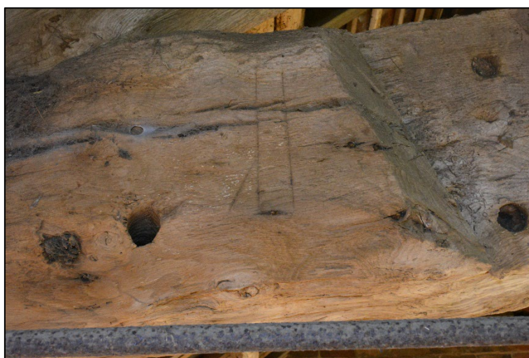
Chiselled carpentry marks on Truss 1, looking east Fig 21
