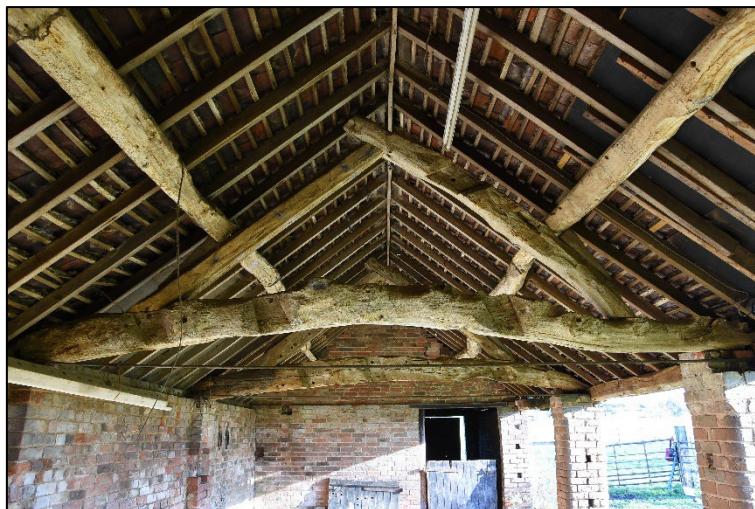
West side of Truss 2, looking east Fig 22
