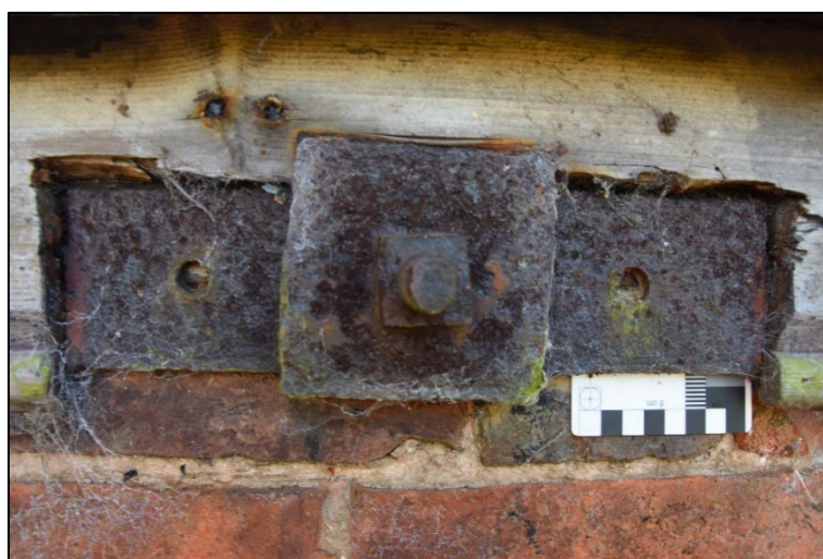
Anchor tie-plate to the north elevation, looking south Fig 12
