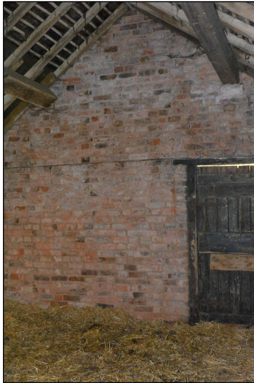
Far eastern room showing brick interior and some of the roof structure, looking east Fig 17
