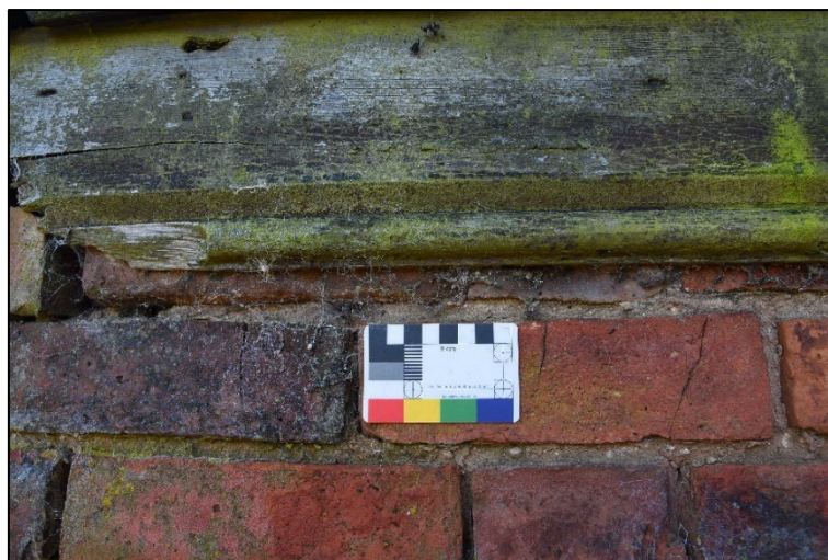
Moulded fascia board to the north elevation, looking south Fig 11
