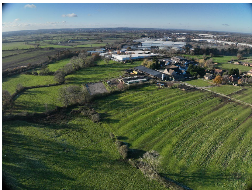
Aerial Photography taken from drone, looking north-west Fig 30
