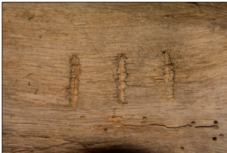
Carpentry marks on Truss 3, looking east Fig 25
