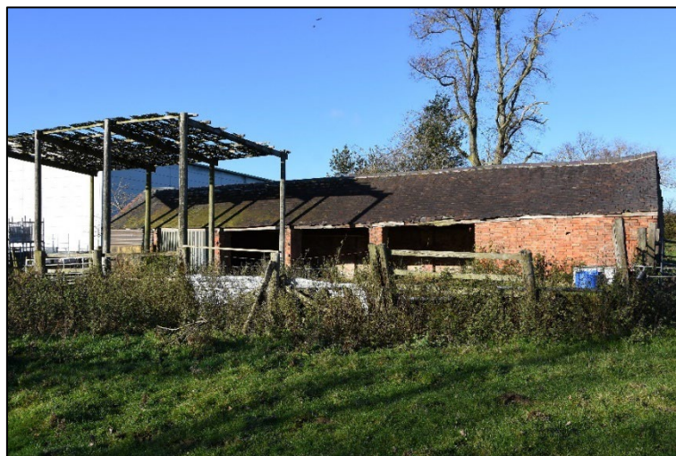
Open-sided south elevation of the building, looking north-west Fig 13
