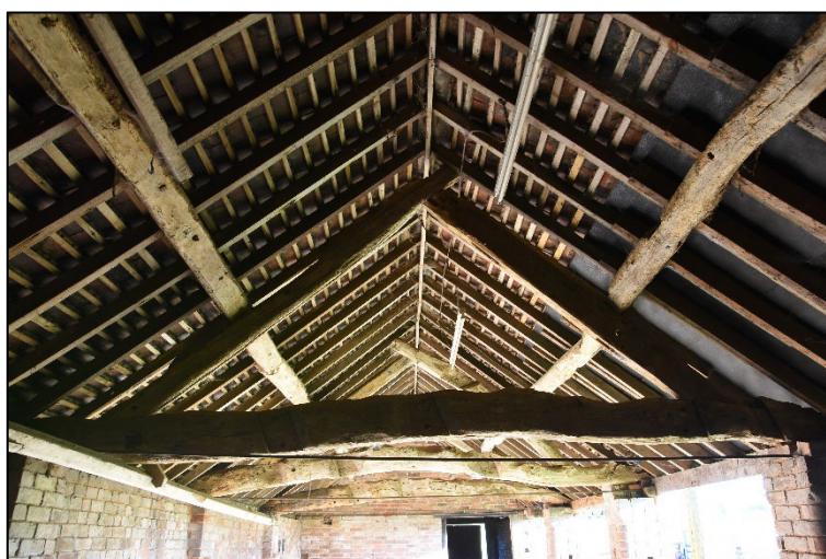
West side of Truss 3, looking east Fig 24
