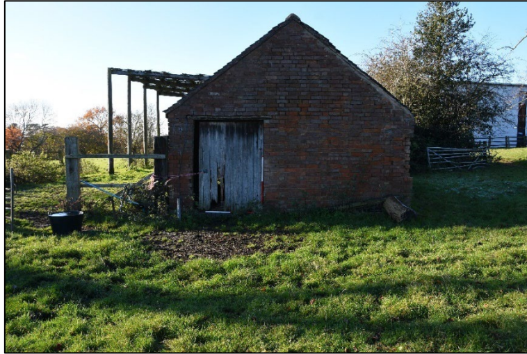
East elevation of the building, looking west Fig 15
