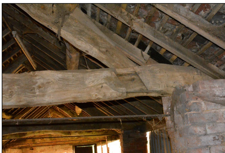
Carpentry marks indicated on Truss 4, looking east Fig 27
