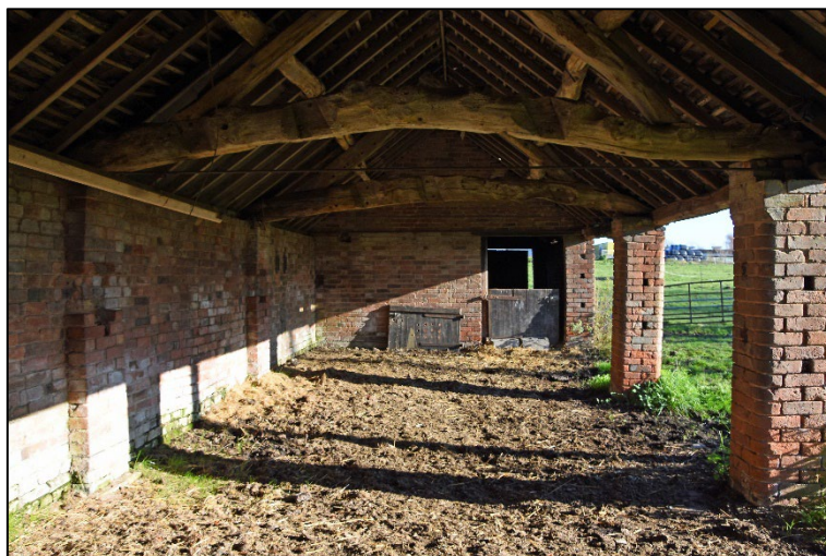
General view of the main space showing brick piers and their mortises, looking east Fig 19
