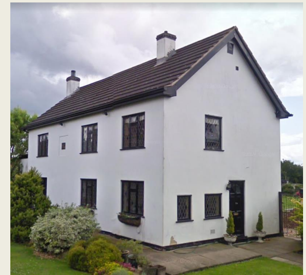
TIDY, BOXED EAVES
