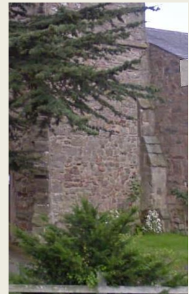
STONE RUBBLE CONSTRUCTION OF THE CHURCH
