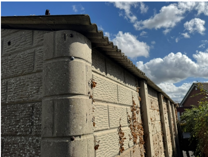
Photo 7: Wall / roof gap
