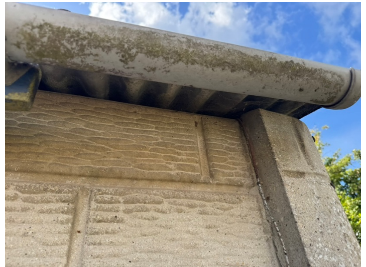
Photo 8: Wall / roof gap
