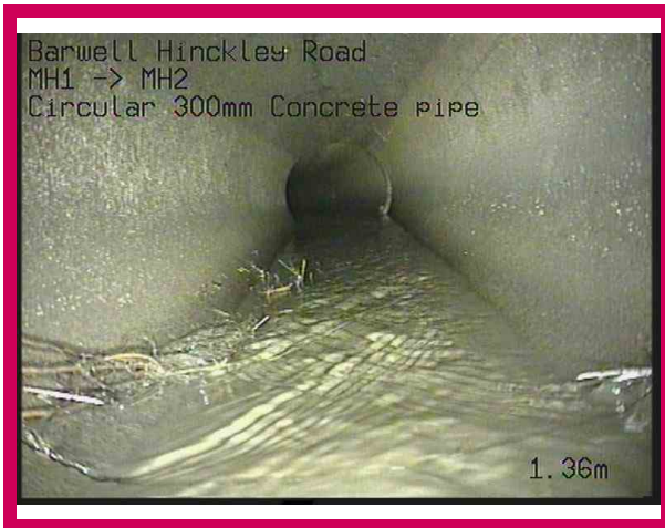
MH1X_be1794be-3572-4021-a4f4-c6ea53cc6a12_20230512_092320_558.jpg, 00:00:14, 1.36 m Roots, fine at joint, start
