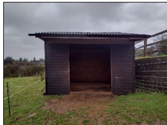
Photograph 25: Field Shelter 'B4'
