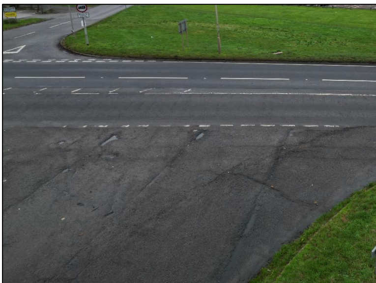
Photograph 6 showing a section of the hardstanding surfaces
