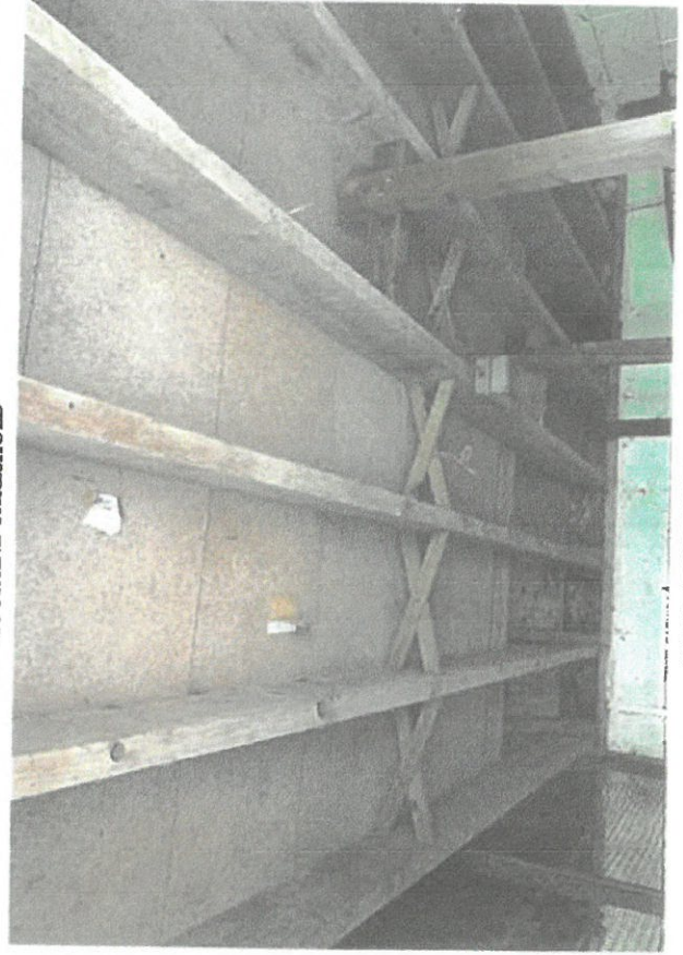
ATTIC FLOOR CONSTRUCTION
