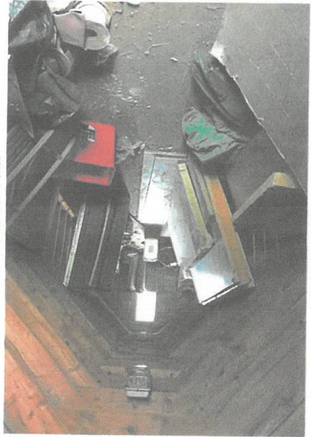
ATTIC LOOKING SOUTH-WEST
