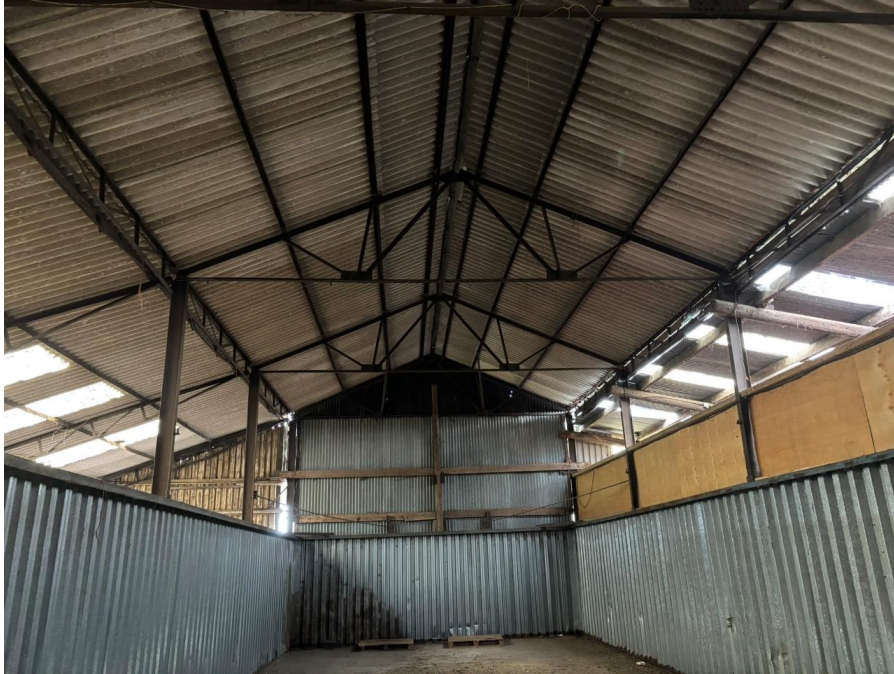
Barn 2 Main Frame Interior
