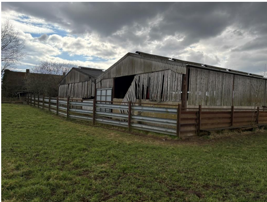
Barn 1 North East Corner
