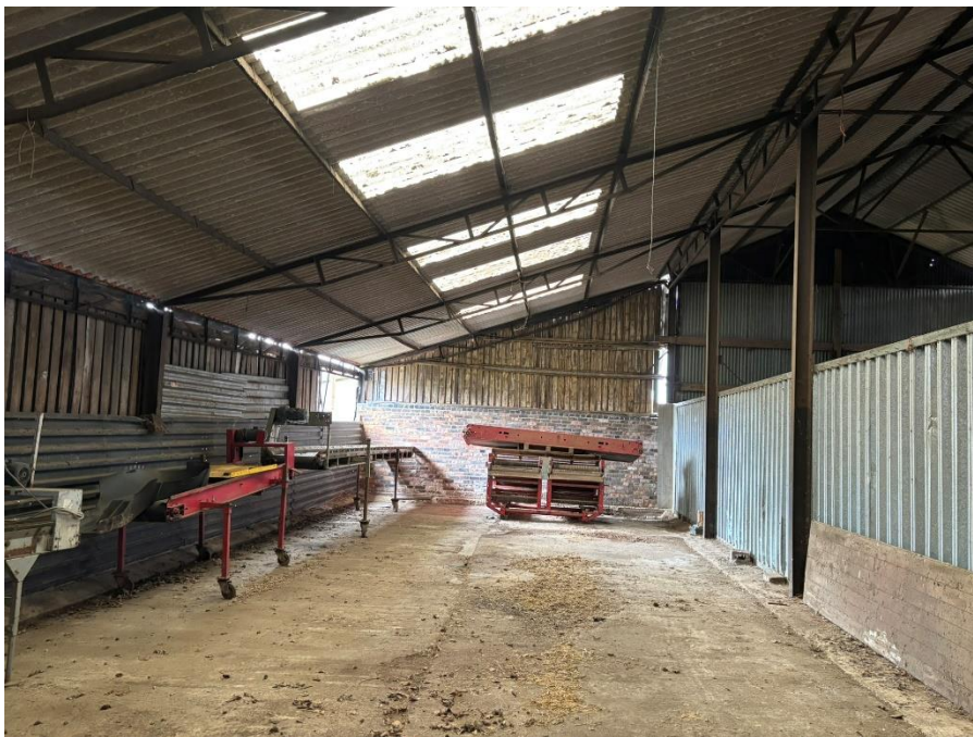
Barn 2 Lean-to Interior
