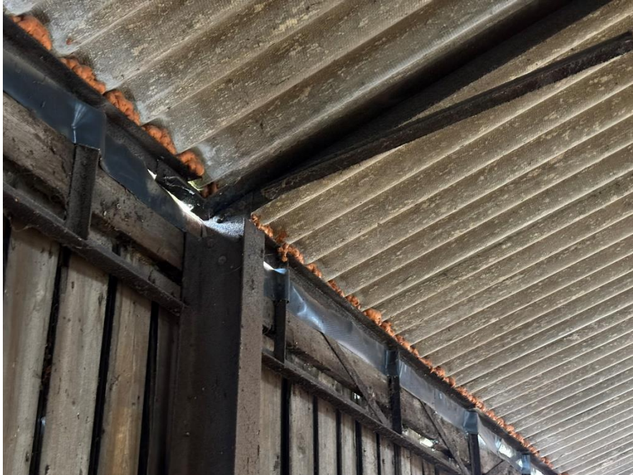
Barn 2 Lean-to Eaves
