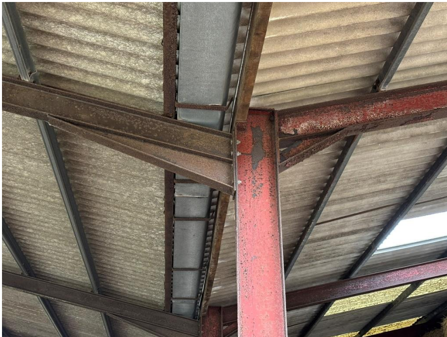
Barn 1 Internal Stanchion
