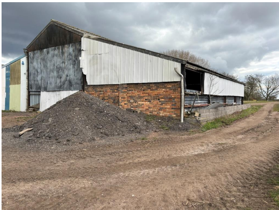
Barn 2 from South West
