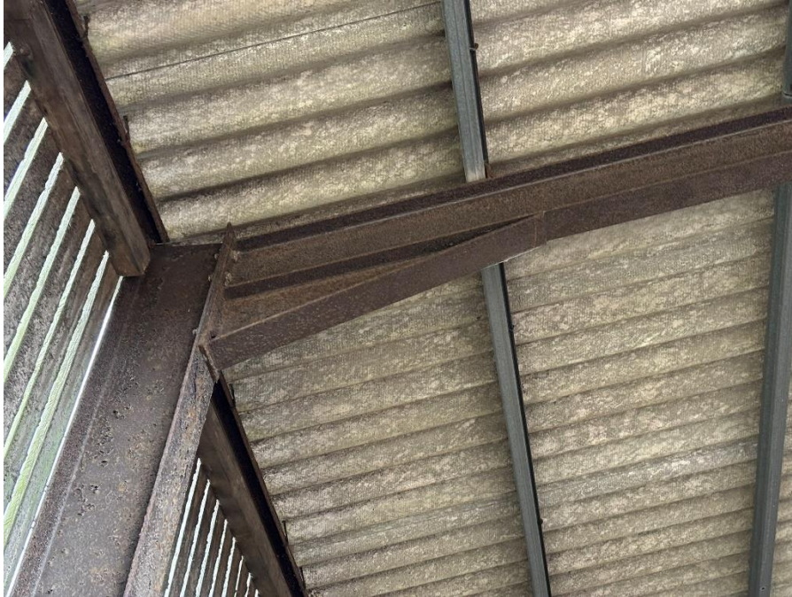
Barn 1 Eaves Haunch
