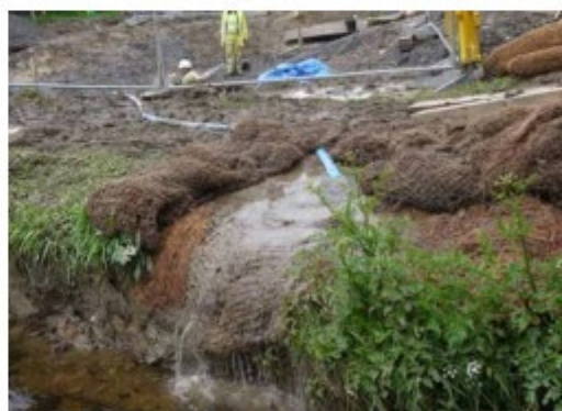
Deployed to treat muddy excavation water
