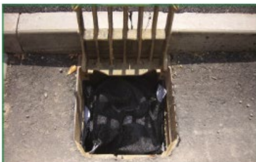
5. Close gully grid.
