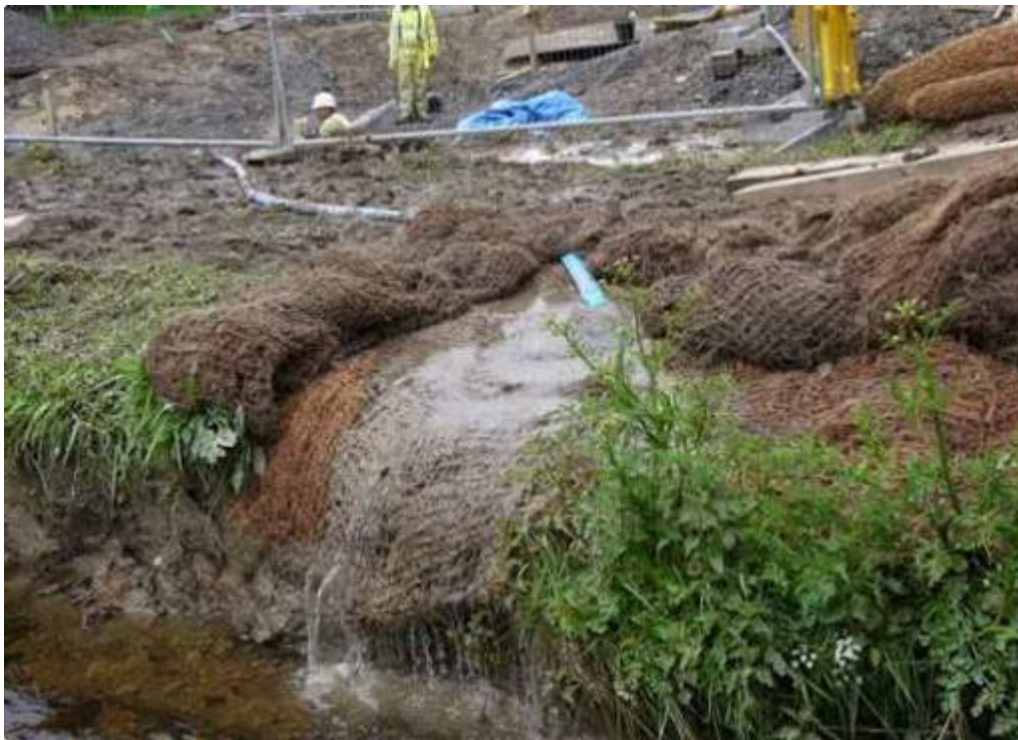
Silt Wattles utilised to separate clean and silty water within a watercourse (image courtesy of Frog Environmental)
