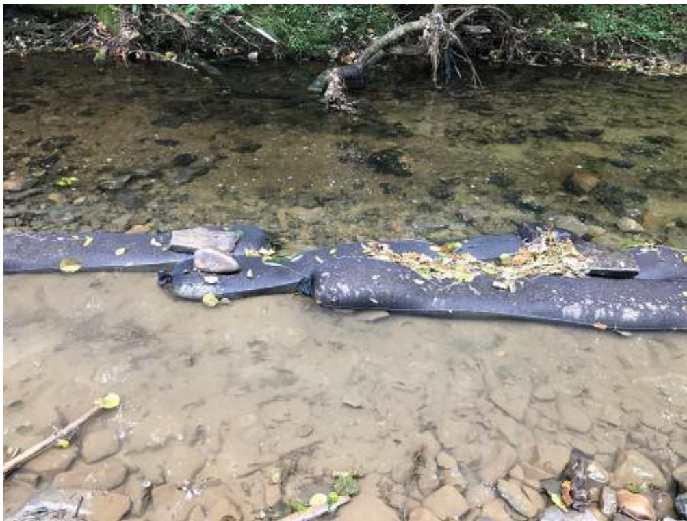
Silt Wattles utilised to intercept silt laden run-off on a road (image courtesy of Frog Environmental)
