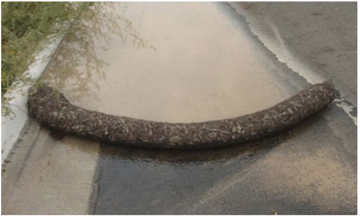
Silt matting and Silt Wattles deployed within a surface watercourse. Silt Wattles create a check dam promoting settlement of suspended solids, which is captured by the silt matting. (image courtesy of Frog Environmental)
