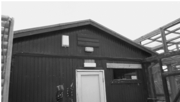
Figure 8.9: Camera to the east of Building 1 – Start of Survey
