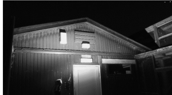
Figure 8.10: Camera to the east of Building 1 – End of Survey
