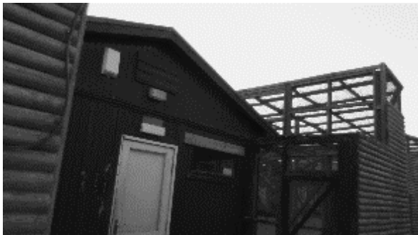
Figure 8.3: Camera to the east of Building 1 – Start of Survey
