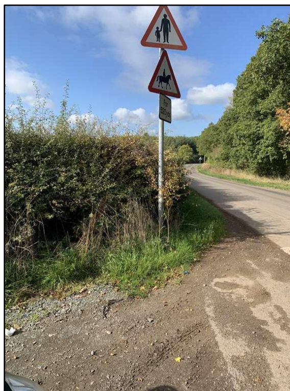
Left hand visibility splay obstructed by hedge and signs
