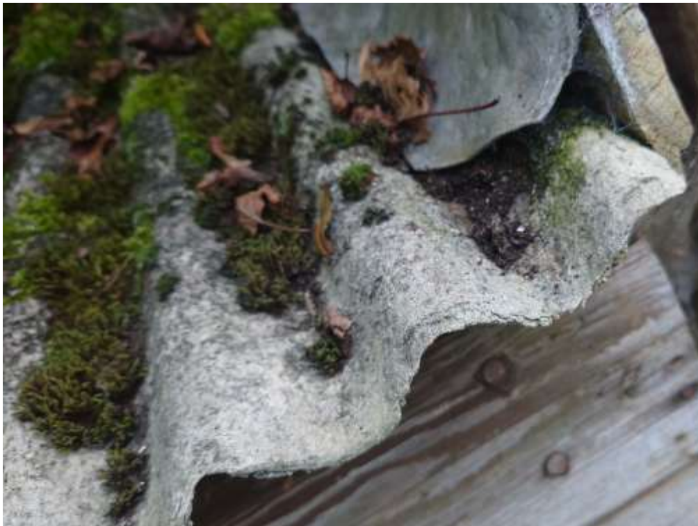
Looking at corrugated cement sheets on roof of structure in field 11
