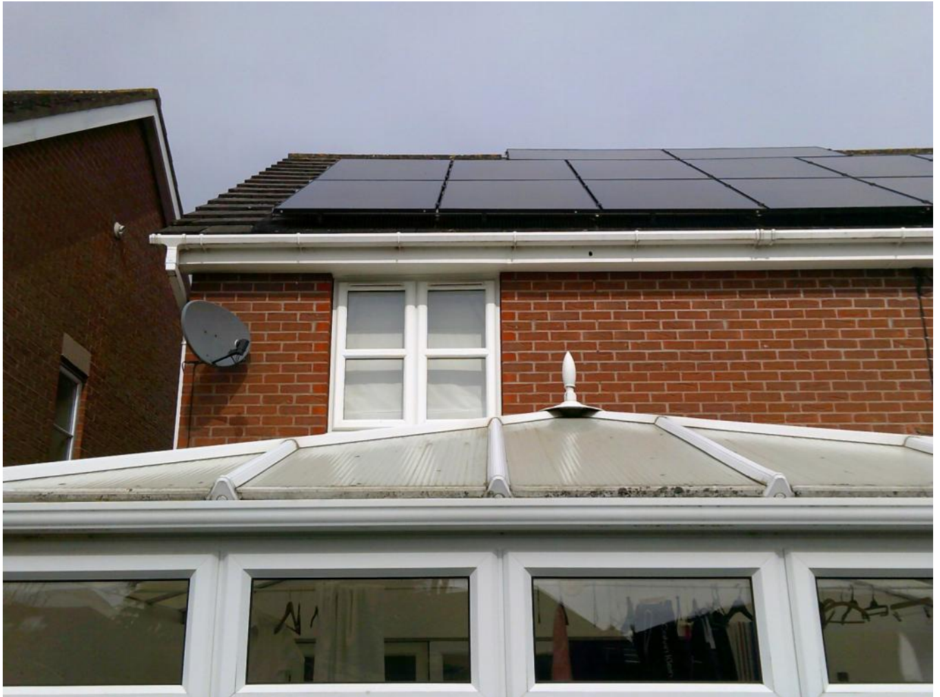
Rear elevation with solar panels
