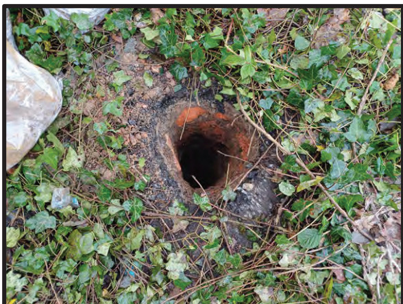
Hand-dug starter pit
