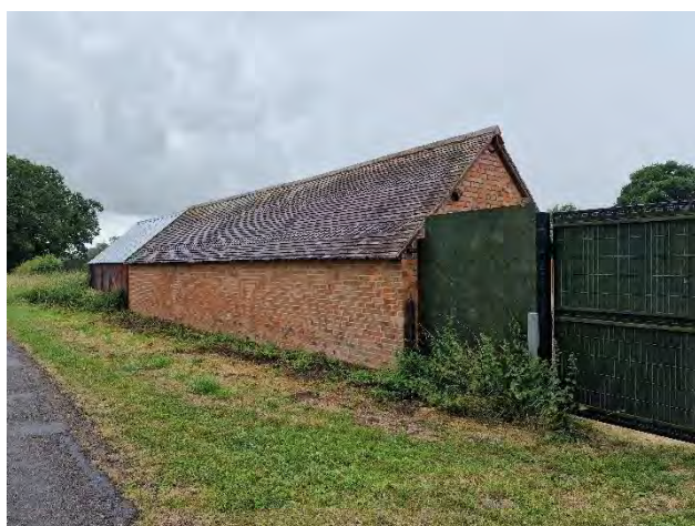
Photo 23: Building B1a, northeast elevation
