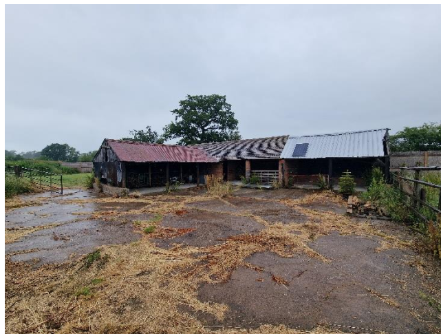
Photo 2: Sealed surface and building on site.
