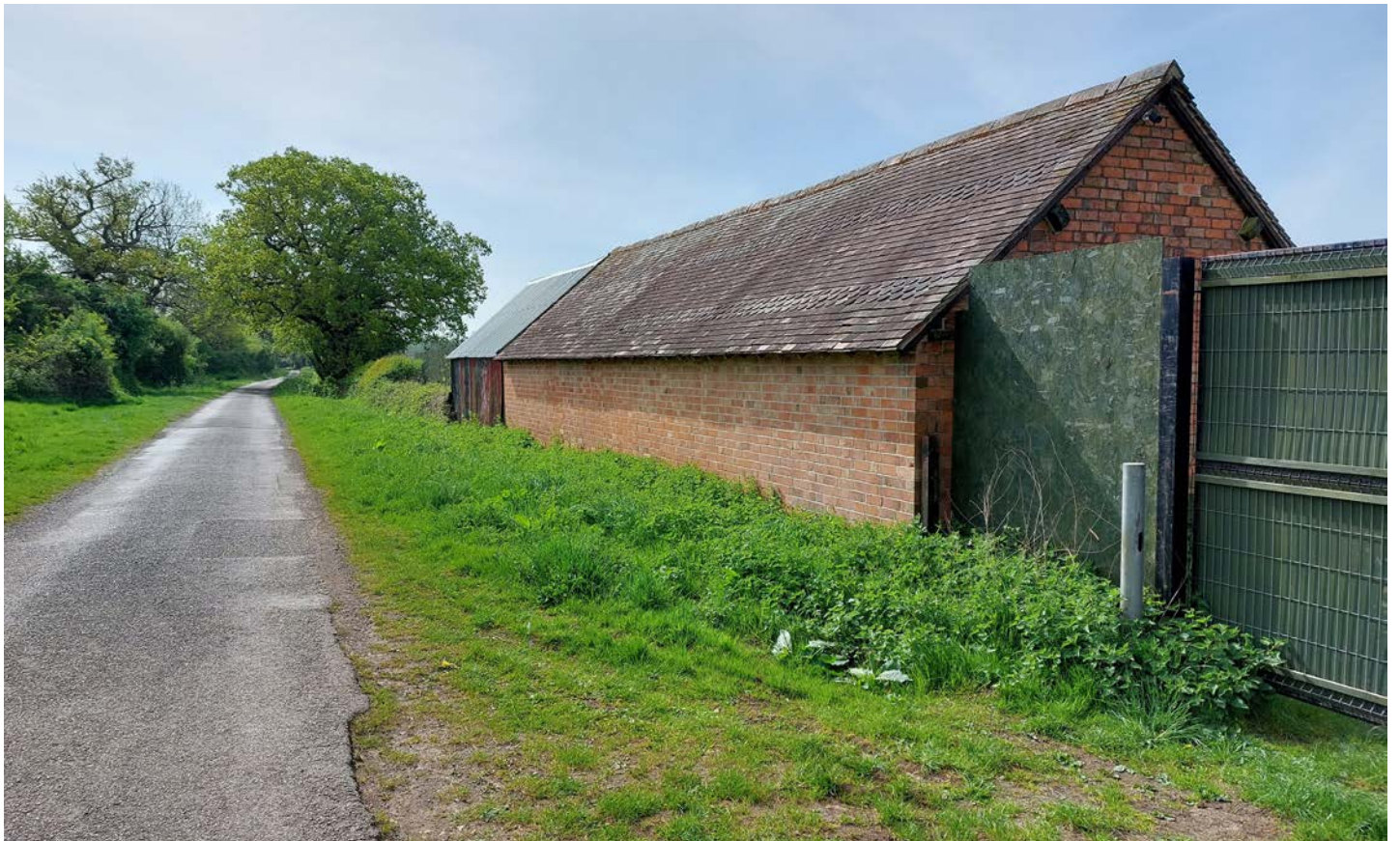
View of existing barn off Sutton Lane looking south-east
