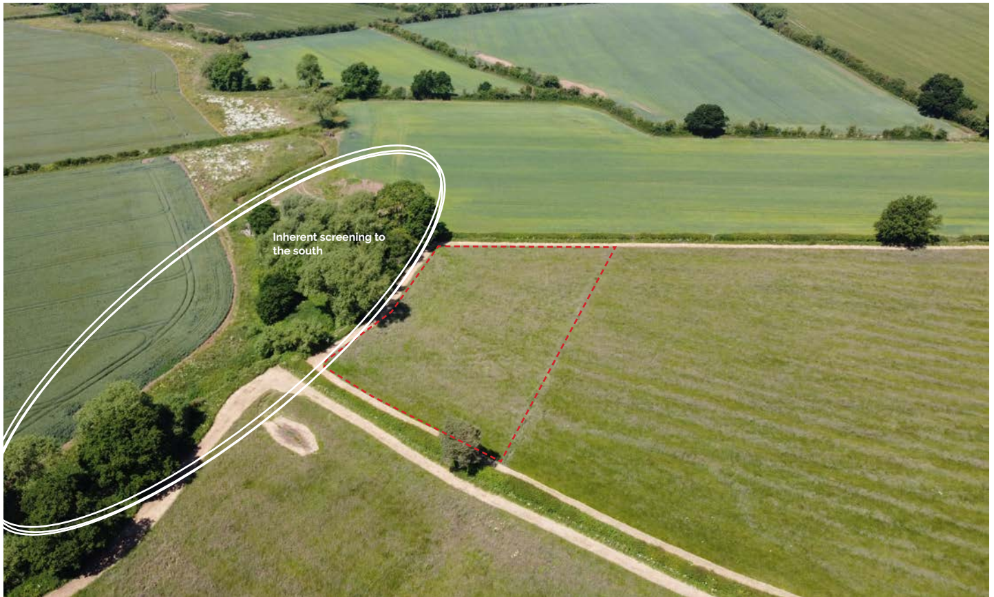
Site of proposed building looking west with view of existing woodland path on site
