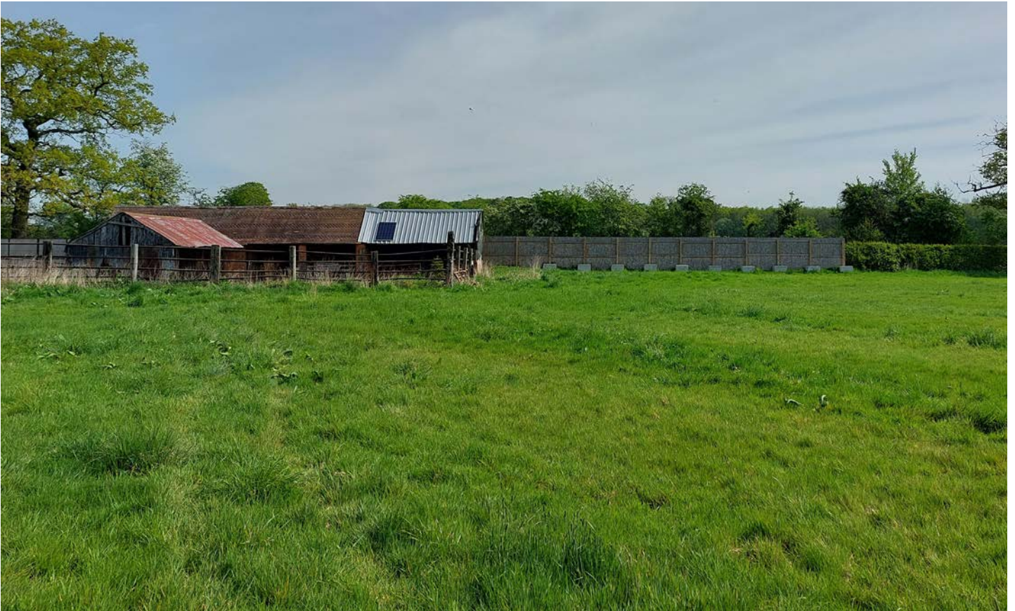
Existing barn - view looking east
