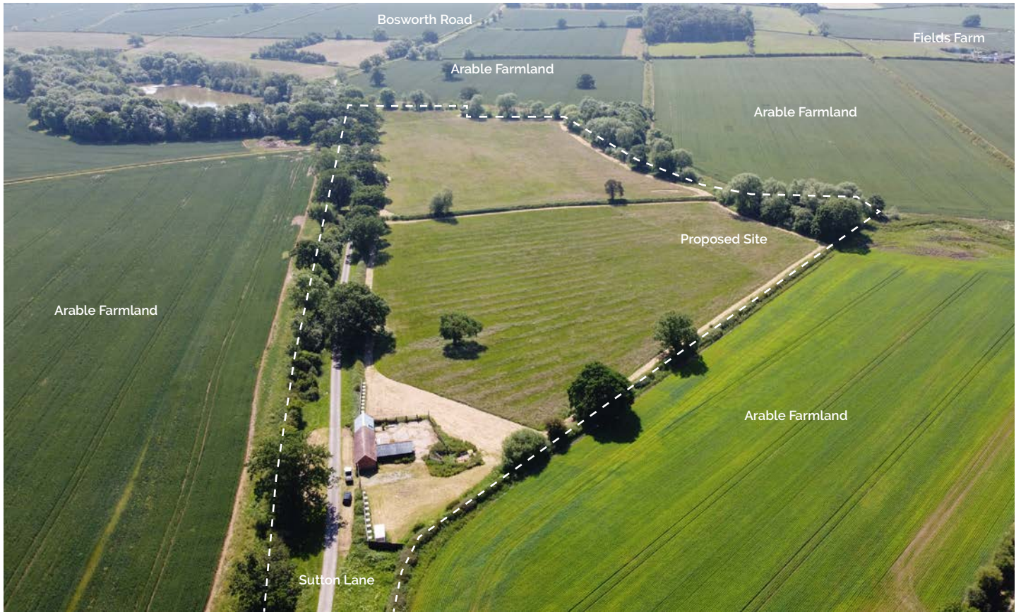
View looking south-east
