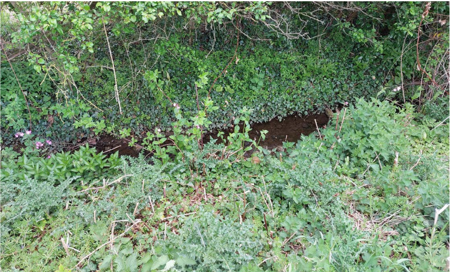
Running ditches on site
