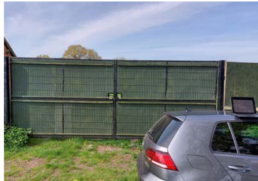
Existing access gates
