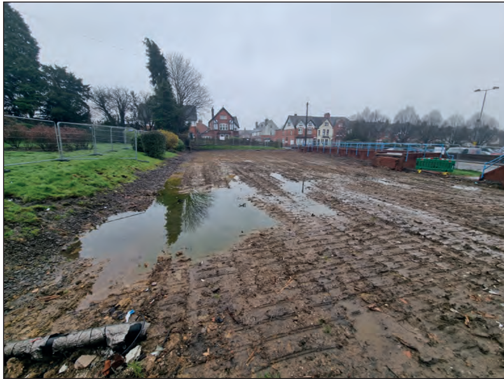
General view of Site, looking south-west
