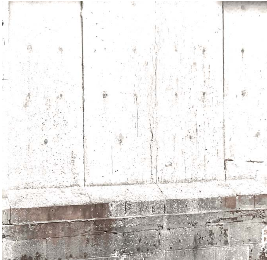
Retaining Wall units/push wall on raised blockwork and slab
