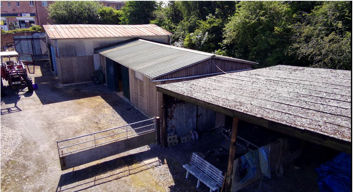
Drone view of buildings
