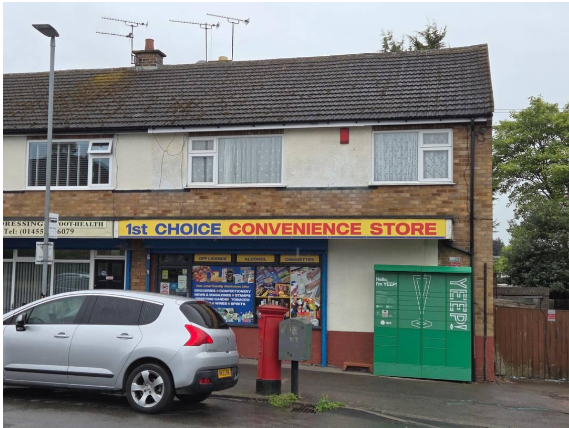
Photograph 1: The northern elevation of the main building.
