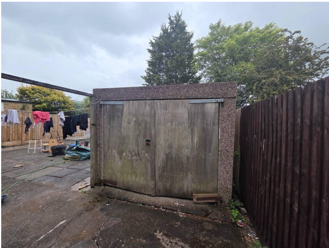
Photograph 4: The northern elevation of Building 2.
