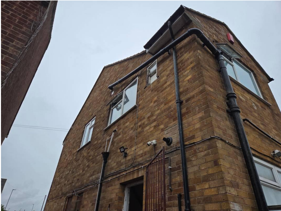
Photograph 3: The eastern elevation of the main building.
