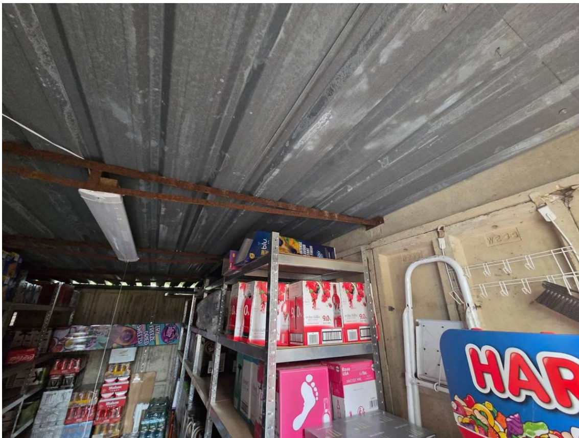
Photograph 6: The view of the internal roof structure – Building 2.
