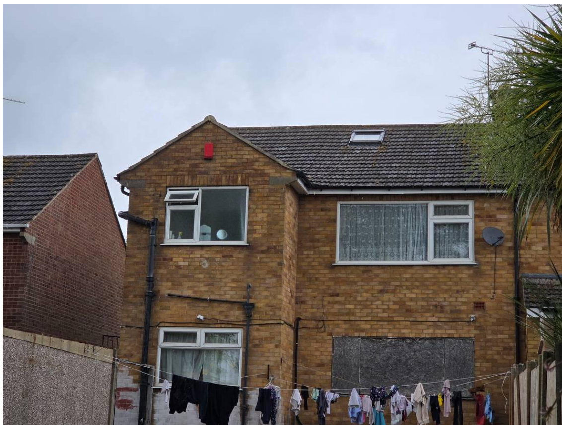
Photograph 2: The southern elevation of the main building.
