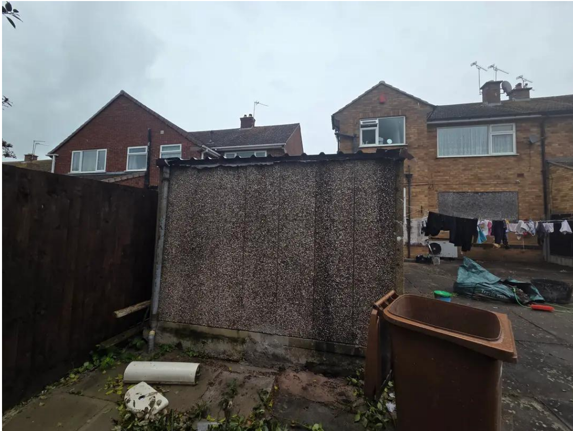
Photograph 5: The southern elevation of Building 2.
