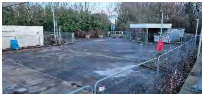
Photo 1: Kiosk and car wash of the PFS, looking southeast.
