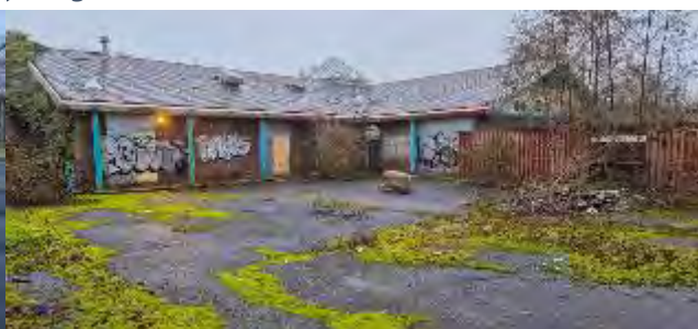
Photo 4: Southeast corner of the services building, facing northwest.
