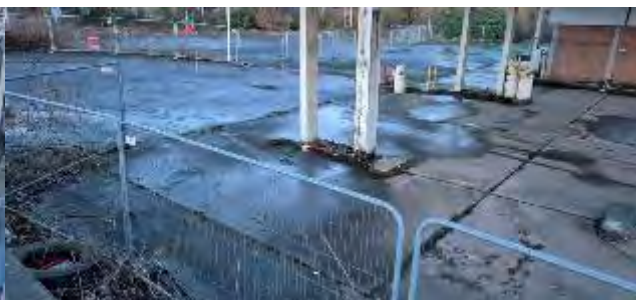
Photo 2: PFS on the east of site, facing northeast.
