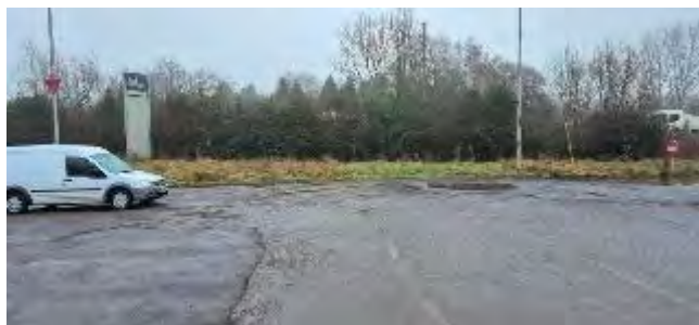
Photo 7: Edge of car park, facing north.
