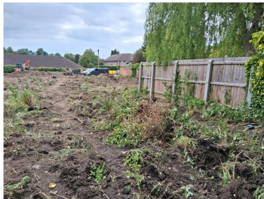
Photo No.6: Facing slightly SW from the north of site showing the general ground conditions occupying site entirety
