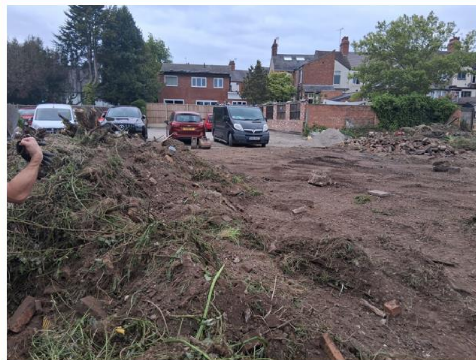
Photo No.2: Facing west from the southern extent of the main site area showing the adj. car-parking area forming SW extent
