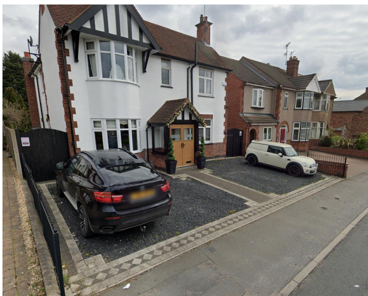
Figure 6 Dwellings with low-level brick walls and mental fencing
