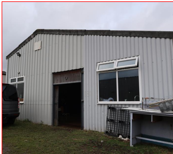
View of barn for re-development
