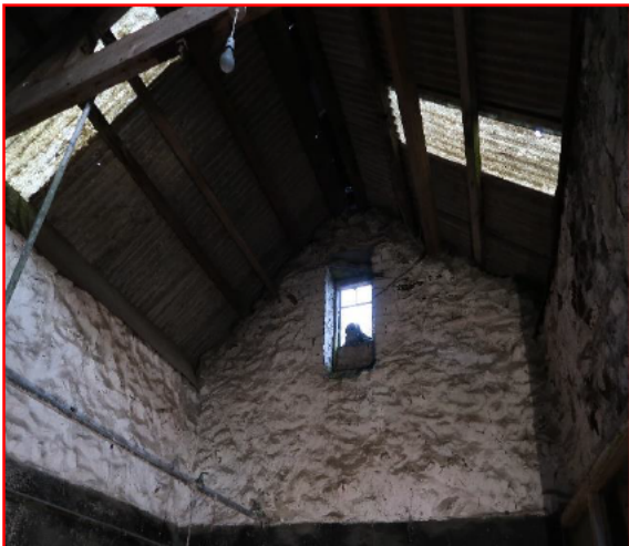
Internal view of barn
