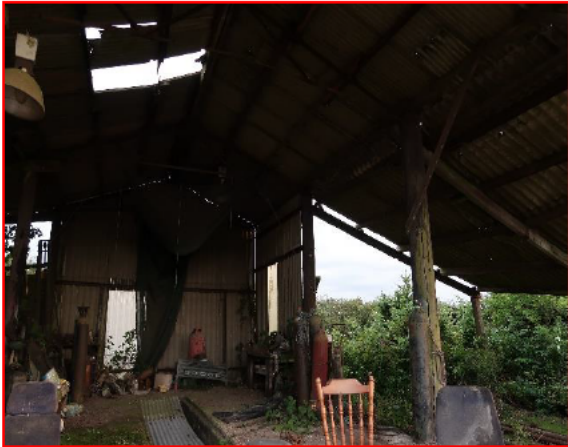
Internal view of barn
