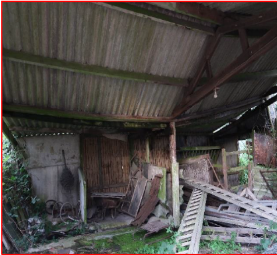
Internal view of barn
