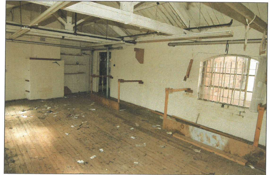
Main building, first floor. Blocked windows on rear wall and inserted doorway. Looking south-west.
