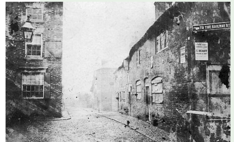
Station Road before demolition
