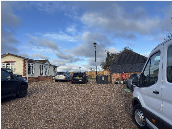
Figure 4: Overview of site.
