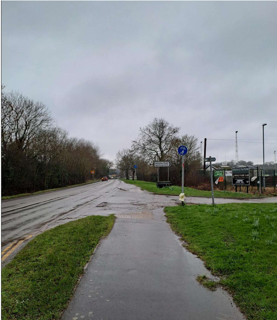
Figure 3.1: Access Road Looking Onto Leicester Road
