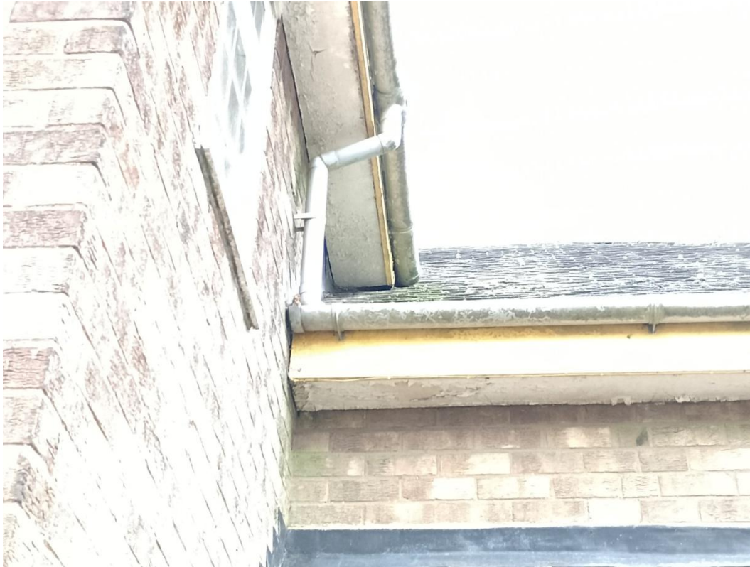
Photo 9: View of gaps at the soffit.
