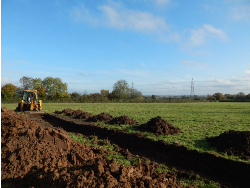
Figure 4: Work in progress on Trench 01, looking east
