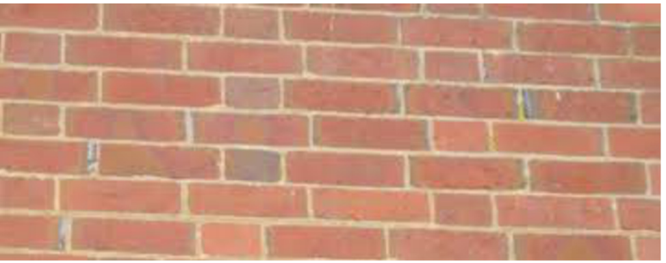
Reclaimed red facing brickwork using Sussex bonding pattern to match neighbouring buildings brickwork
