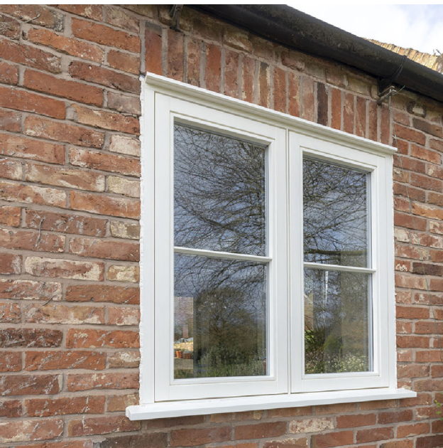
White painted timber windows to house facing elevation
