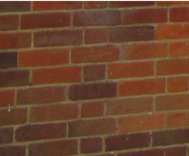
Existing red facing brickwork
