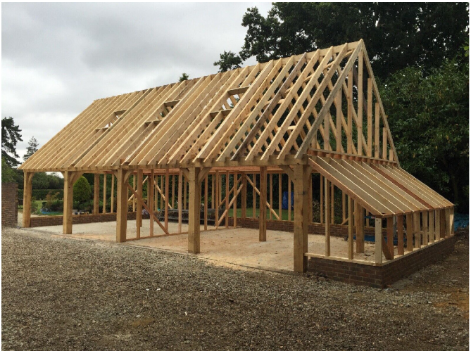
Oak frame structure to car port
