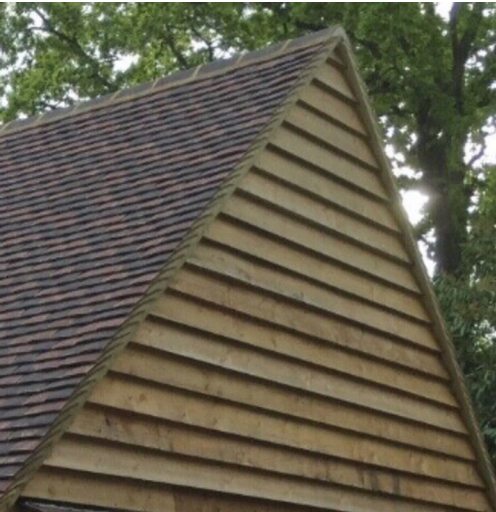
Timber cladding to car port
