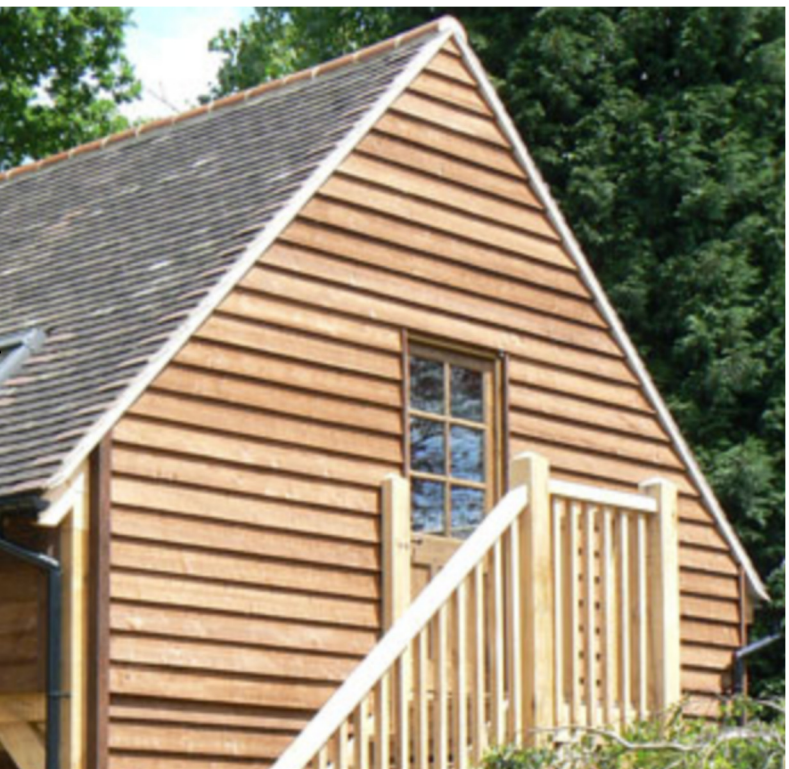
Timber stairs & timber door to studio over car port
