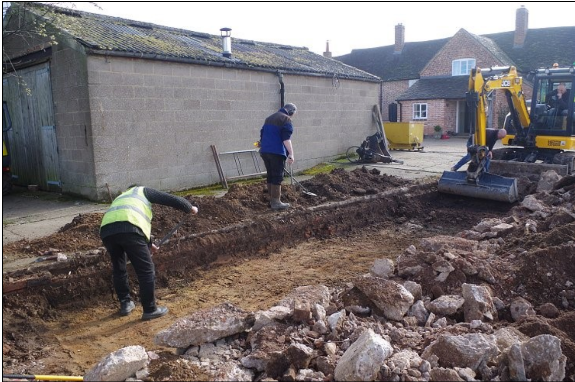
Photo 3. Trench 1, looking SE. Cleaning of trench and metal detecting in progress.
