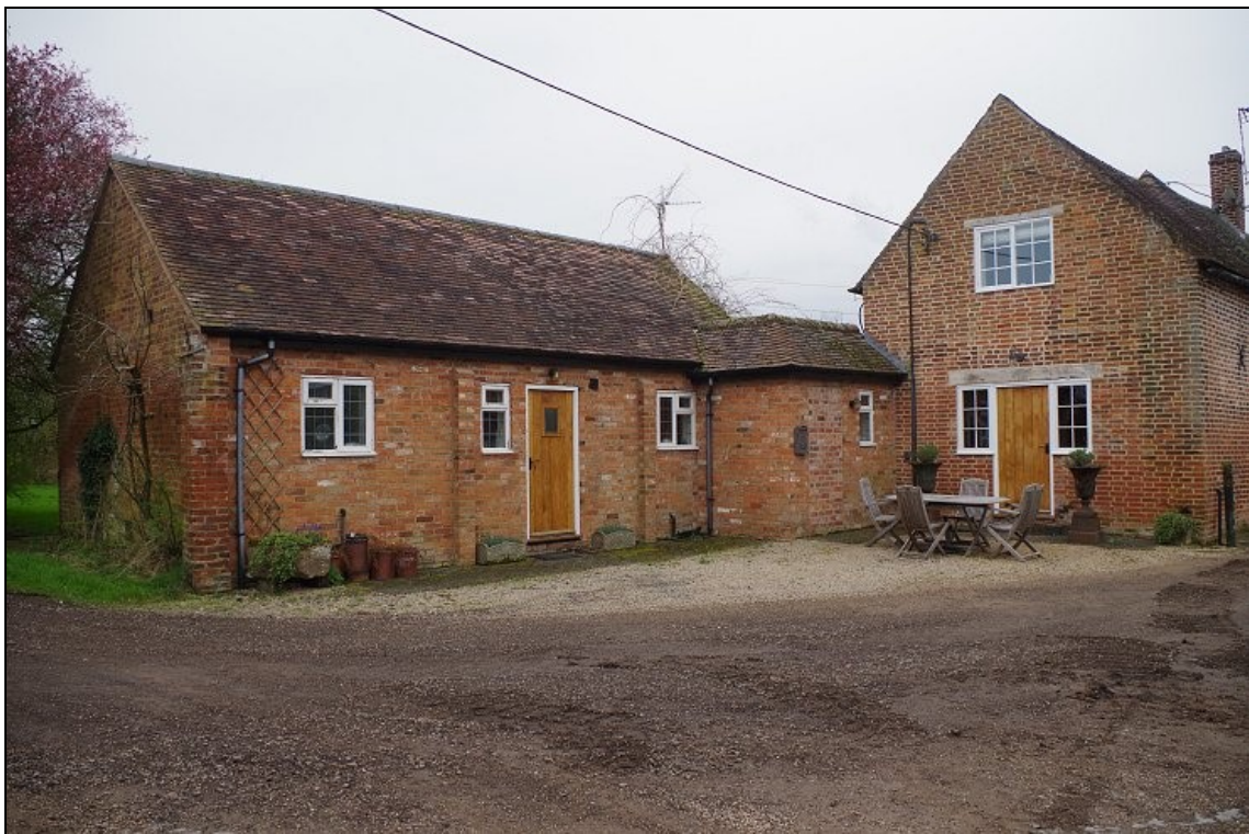
Photo 20. Area of proposed Trench D, not excavated due to live drains running across this area from house and annexe to septic tank in vicinity of proposed Trench F, looking S.
