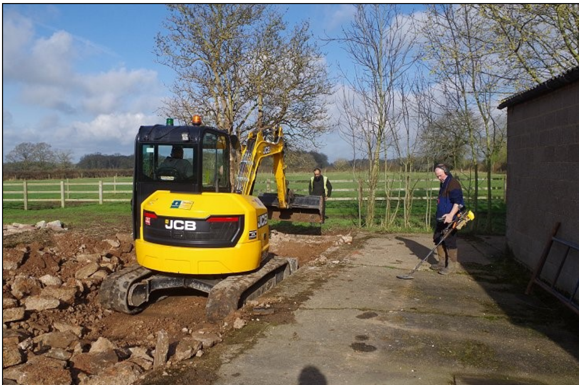
Photo 2. Excavation of Trench 1 in progress, following removal of concrete slab, looking NW.
