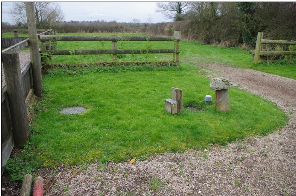
Photo 22. Area of proposed Trench F, not excavated due to location of live septic tank (note inspection chamber cover), looking SE.
