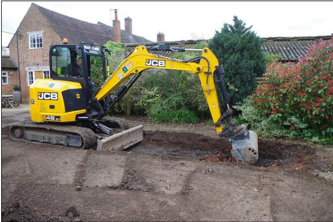
Photo 17. Excavation of Trench 4 in progress, looking S.
