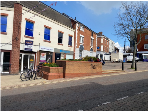
Photo 1: Raised Planters on the Market Place.
