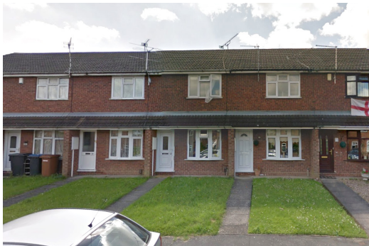
6 - Two-storey terraced houses
