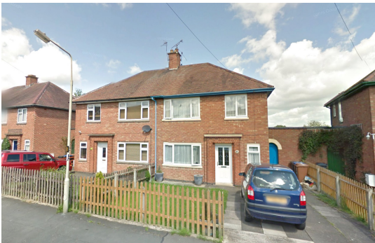
2 - Two storey semi-detached houses
