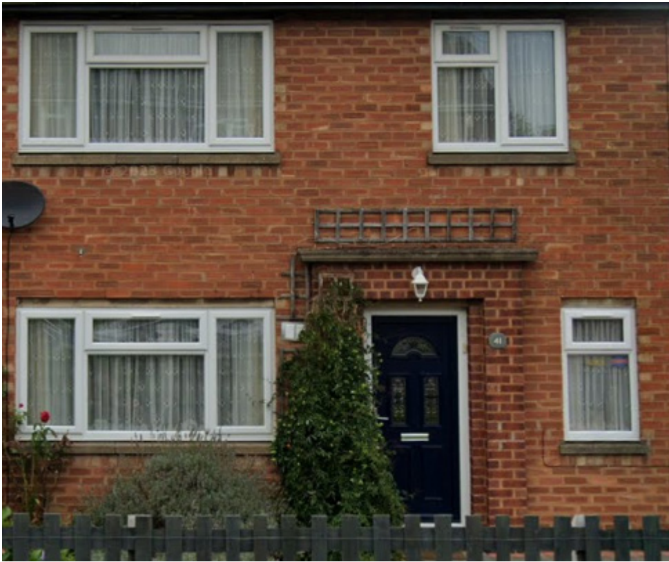
Red brick and UPVC windows
