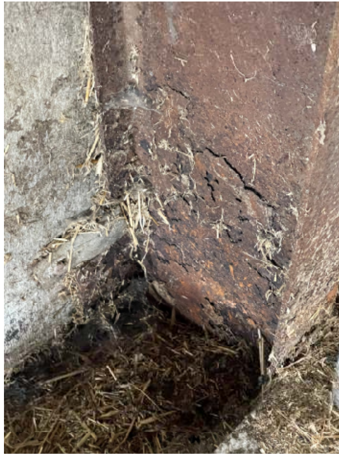
Figure 10: Delaminated column
