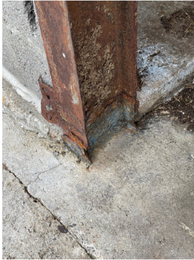
Figure12: Base of gable post
