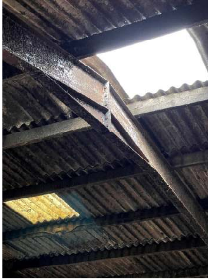
Figure 8: Portal frame ridge connection
