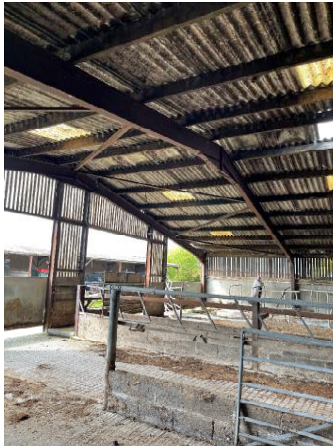
Figure 16: Roof bracing and gable posts
