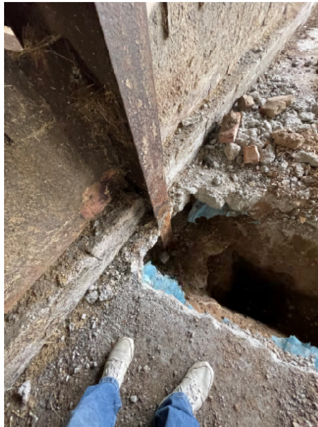
Figure 5: Internal trial hole
