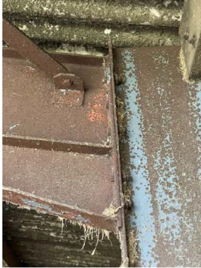
Figure 7: Portal frame eaves connection
