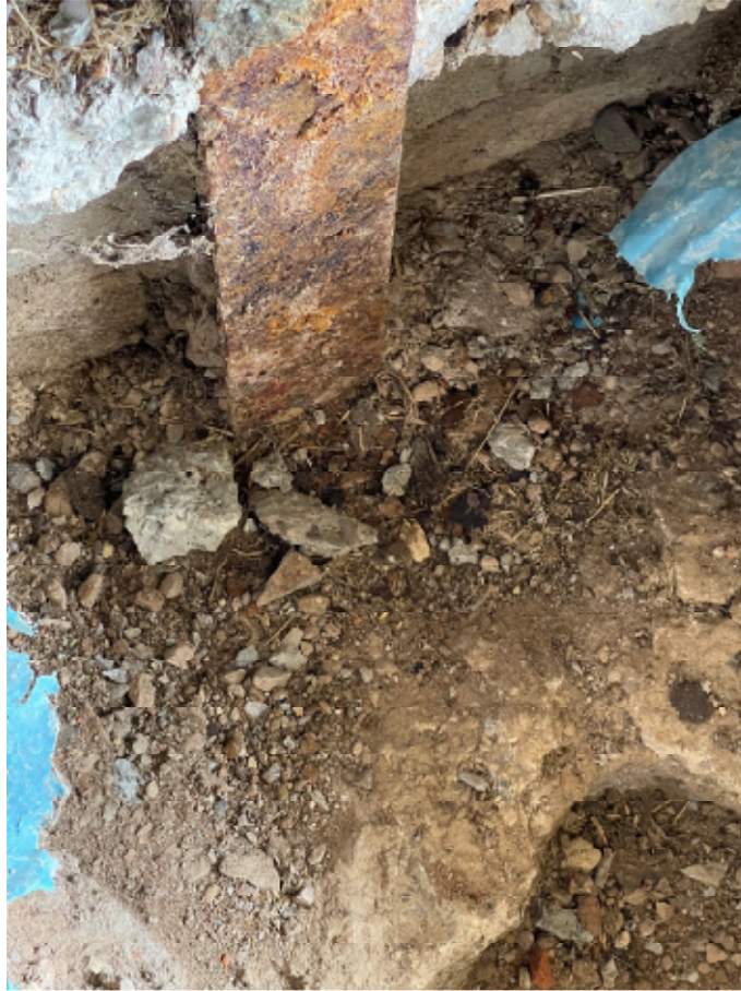
Figure 15: Column pocket base
