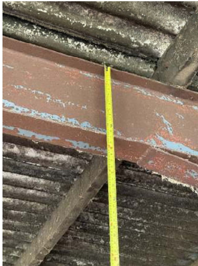
Figure 6: Portal frame rafter
