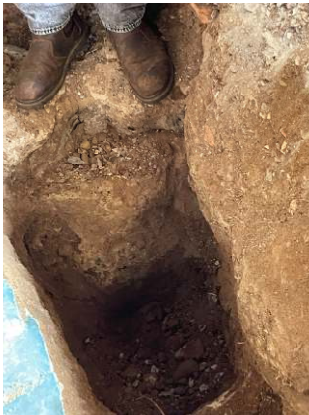
Figure 4: Foundation trial hole
