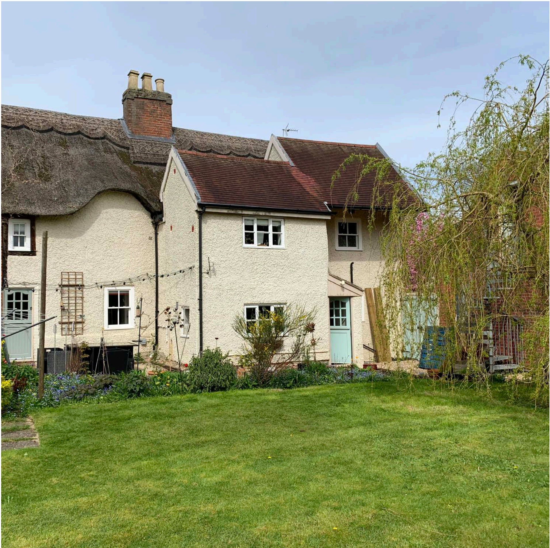
Above: Photograph of the rear roof of the garage Right: Photograph showing the rear elevation of the property
