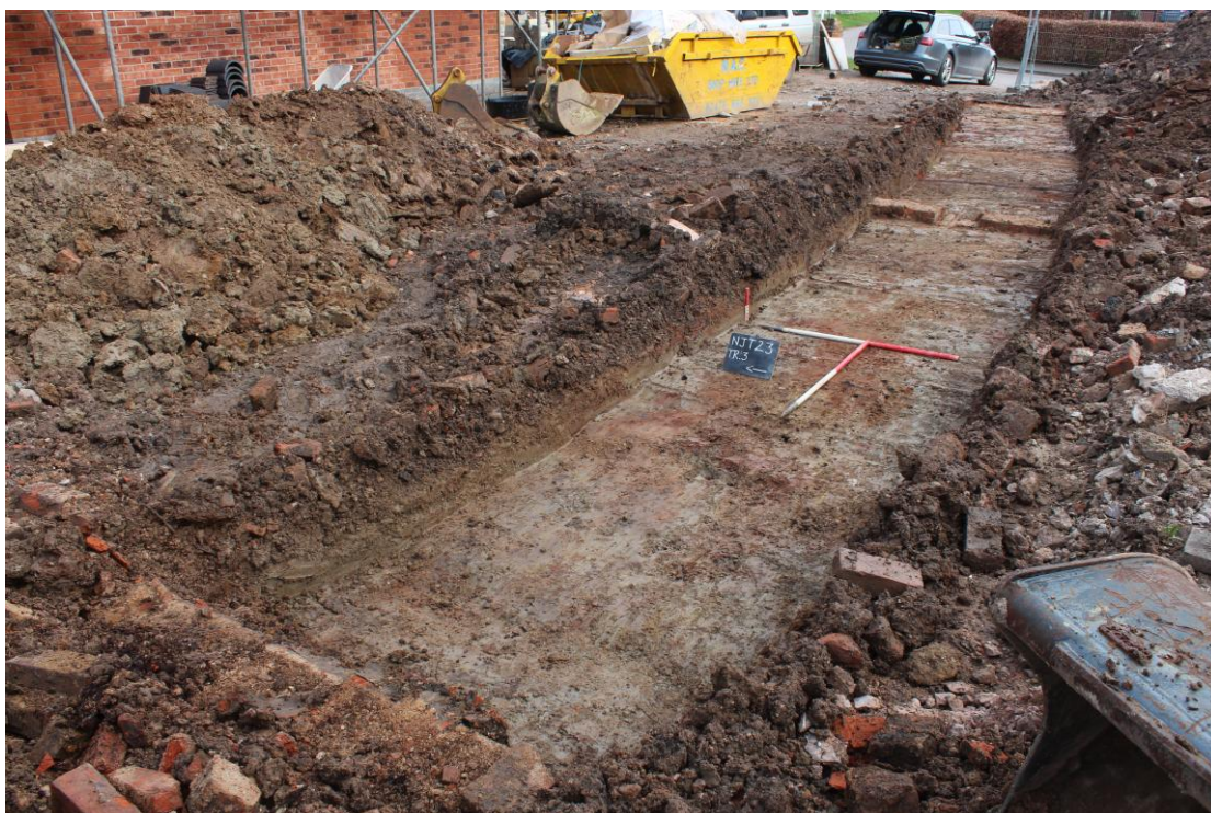
Plate 15; trench 3, view northeast.
