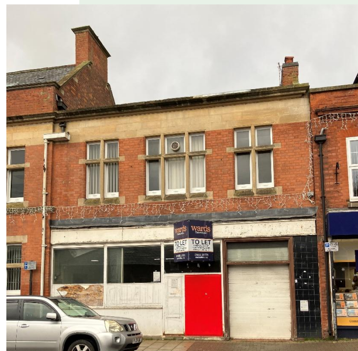
The post office counter shopfront now
