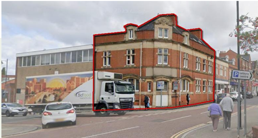
The Existing Building
