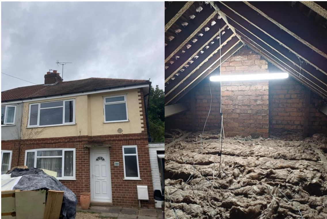
Photograph 2 & 3: The south elevation of the building and view of the internal roof structure.
