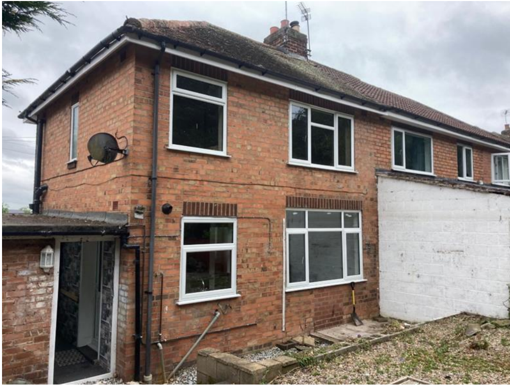
Photograph 1: The north elevation of the building and garage.
