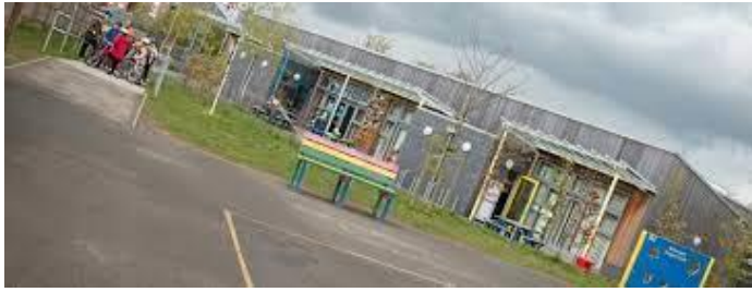
Block D – Cedar Cladding
